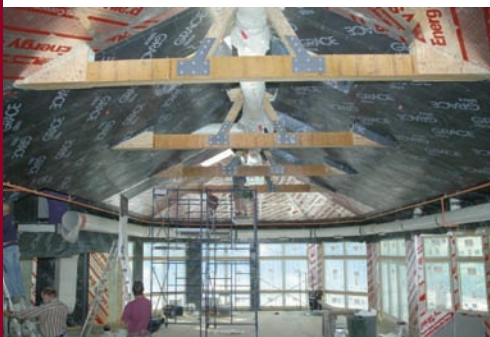
Vaulted ceiling assembly being installed
