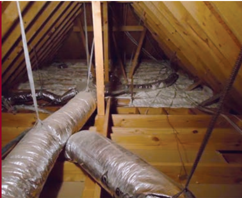
Open cell foam being installed
