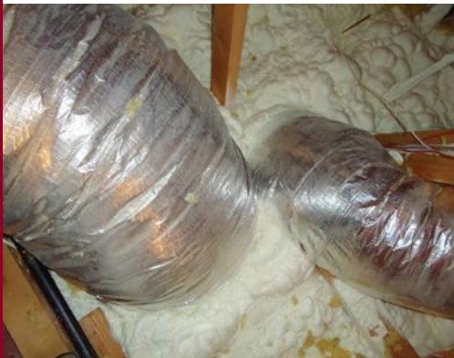
Spray foam seals open duct chases
