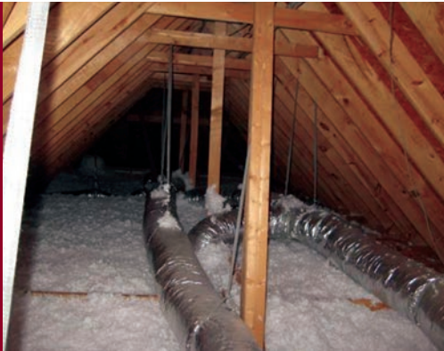
Attic complete after blown-in fiberglass install
