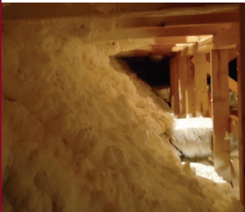
Spray foam fixes open flooring system
